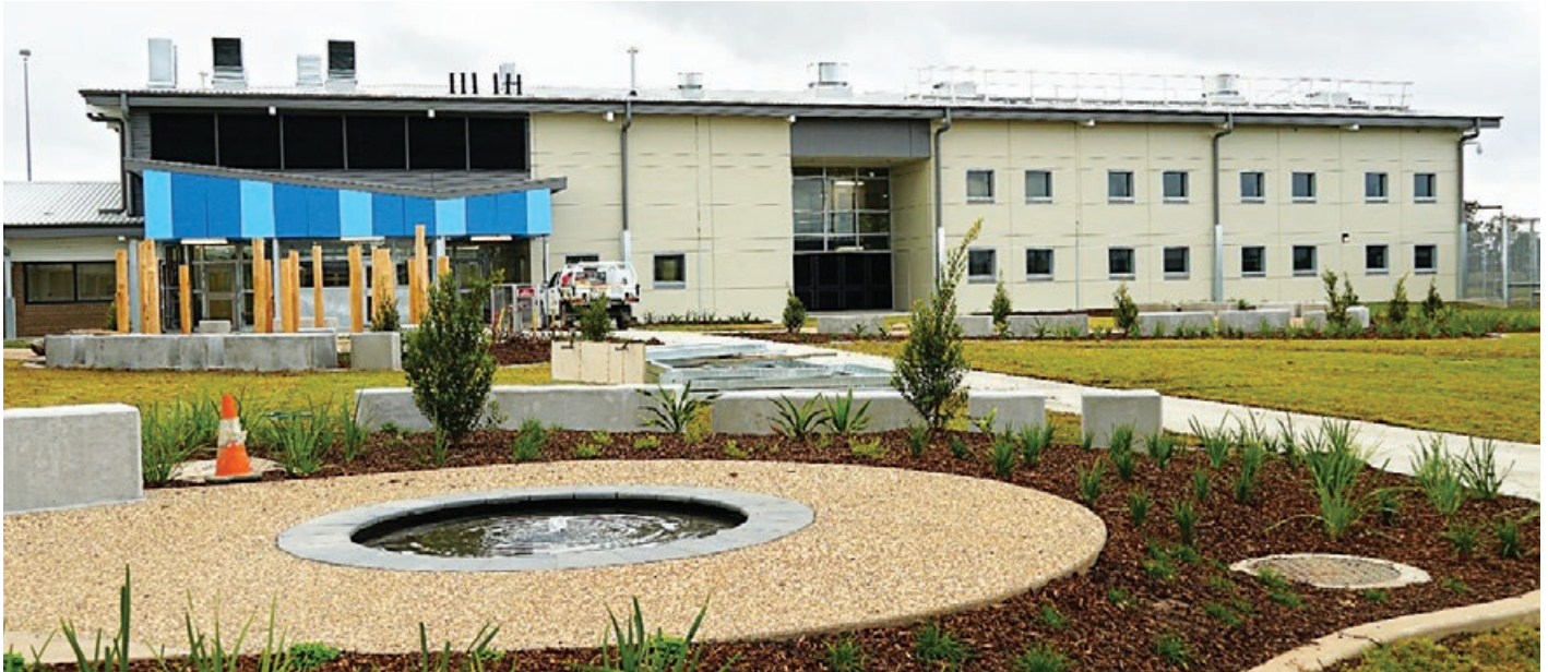
The newly completed 102-bed accommodation block at Fulham Correctional Centre.
