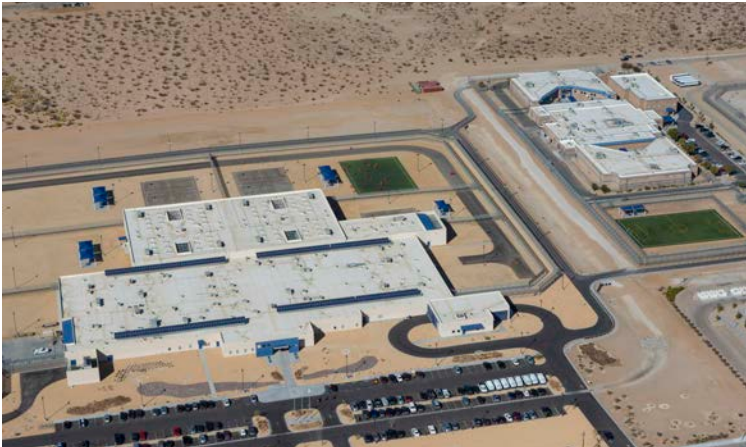
Adelanto Detention Facility
