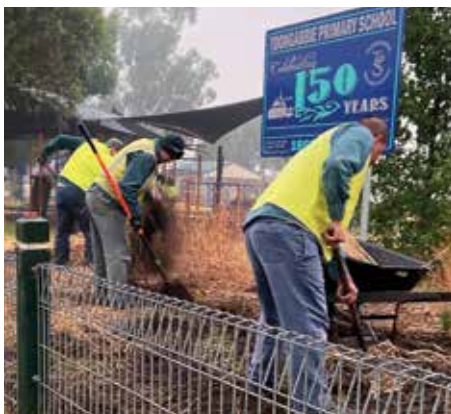
Fulham work crews are always in high demand.
