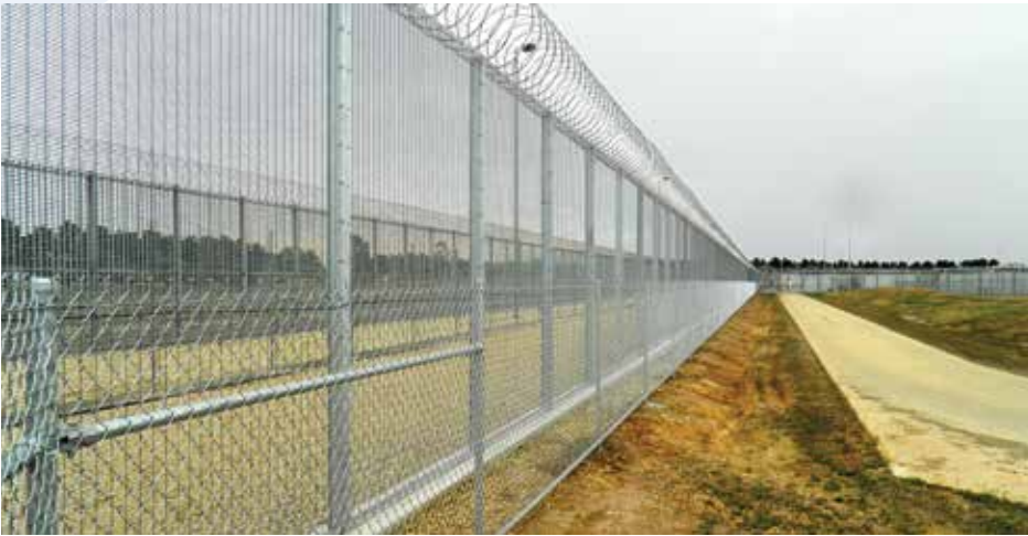
A section of the new inner perimeter fence being constructed at Fulham Correctional Centre.
