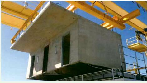
A standard two-cell unit. The door in the middle allows access to services such as power and water.
